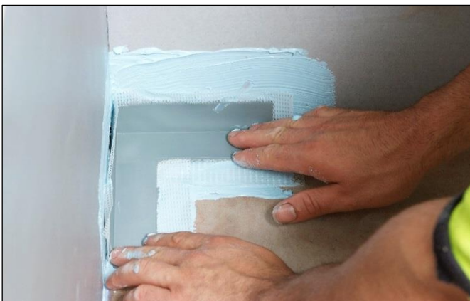
Installing Elastoproof Prefabricated Corners
